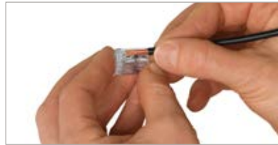
Strip conductor to 11 mm.
